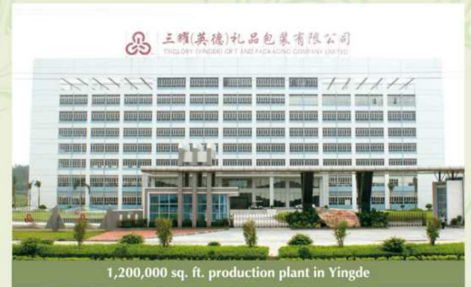
1,200,000 sq. ft. production plant in Yingde
